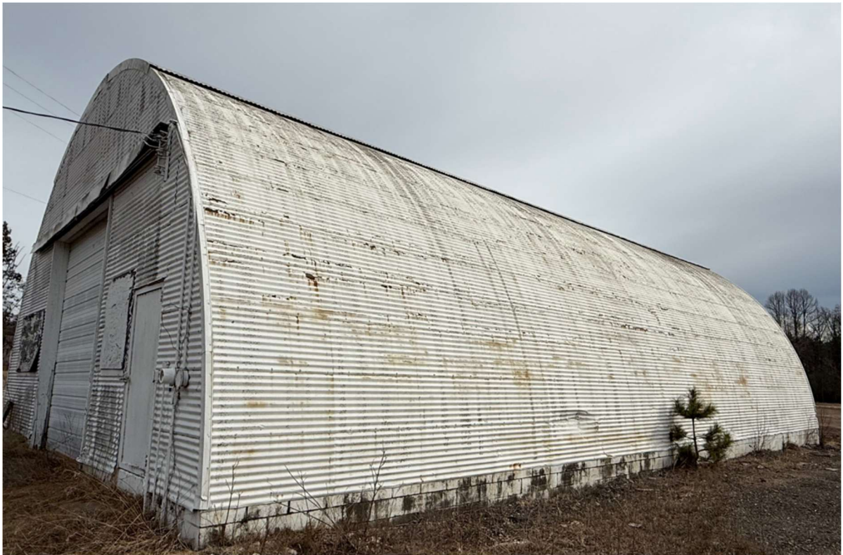
“Quonset Hut” Removal by May 31,2025
